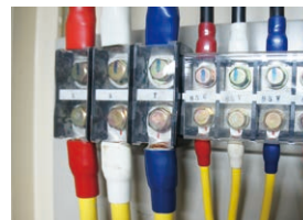
Locations with covered terminals
