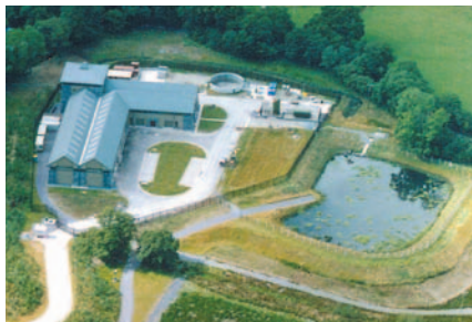
Example of remote pumping station.
