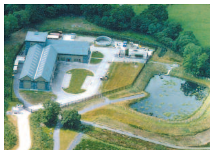
Example of remote pumping station.
