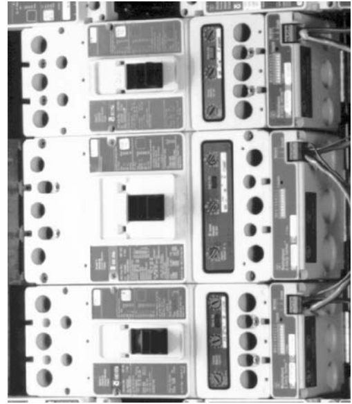
Series C Breakers with Energy Sentinel
